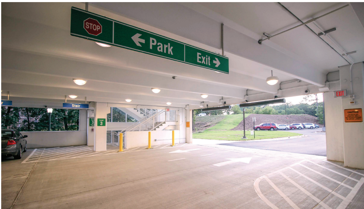
Figure 1.1. Well-maintained parking structures provide a user-friendly atmosphere. Photo: University of Mississippi.
